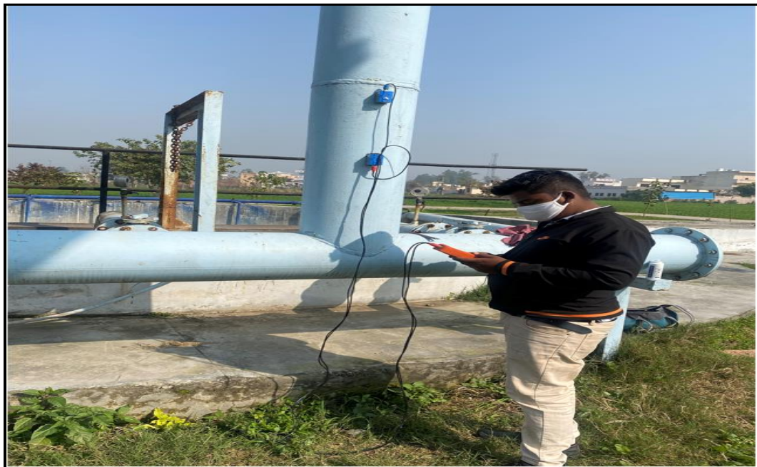
Figure: - Flow Measurement on STP primary Pump
