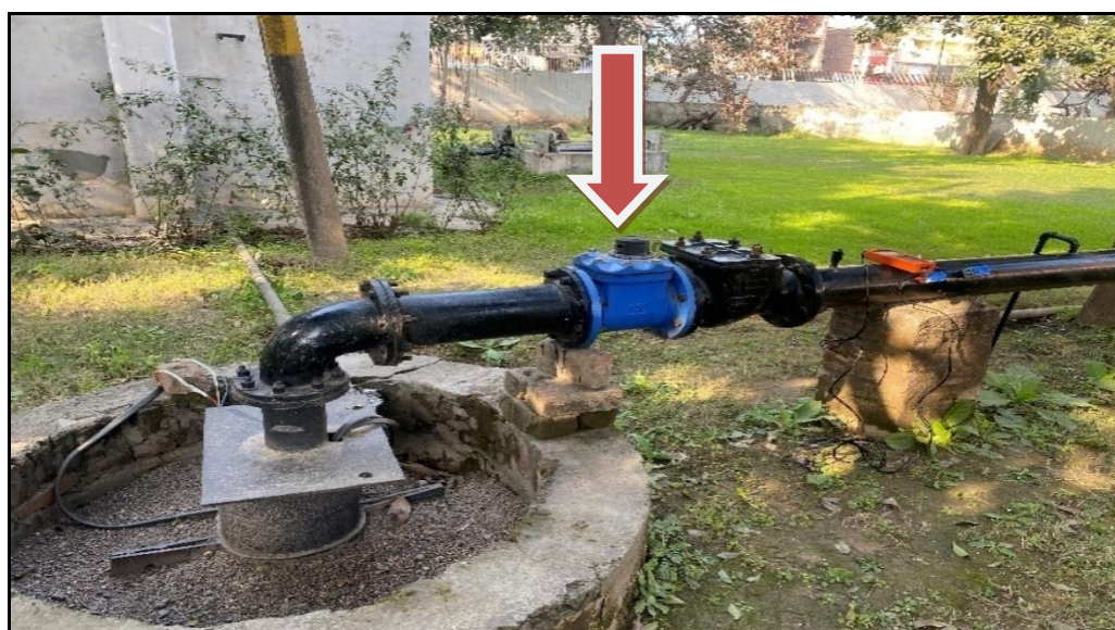
Figure: -2.1 fresh water supply from Borewell for University campus
