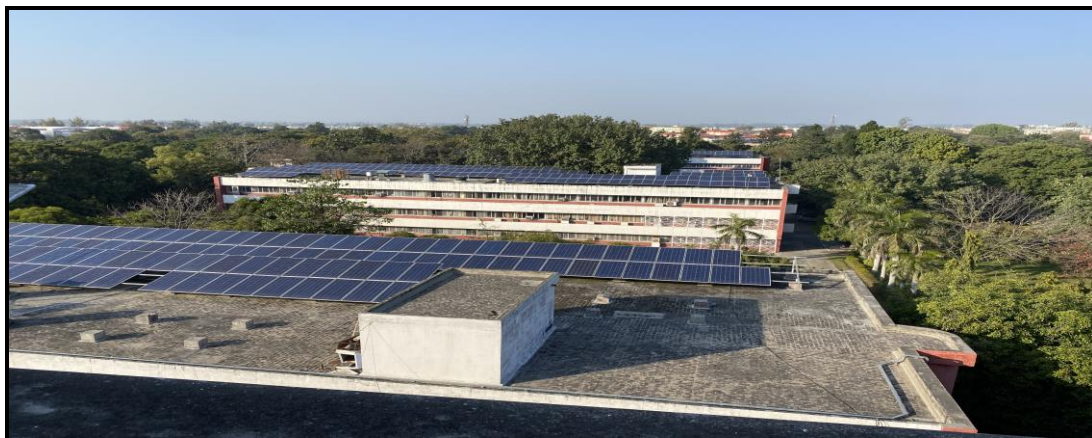
Solar Module (Panel) at Different Buildings
