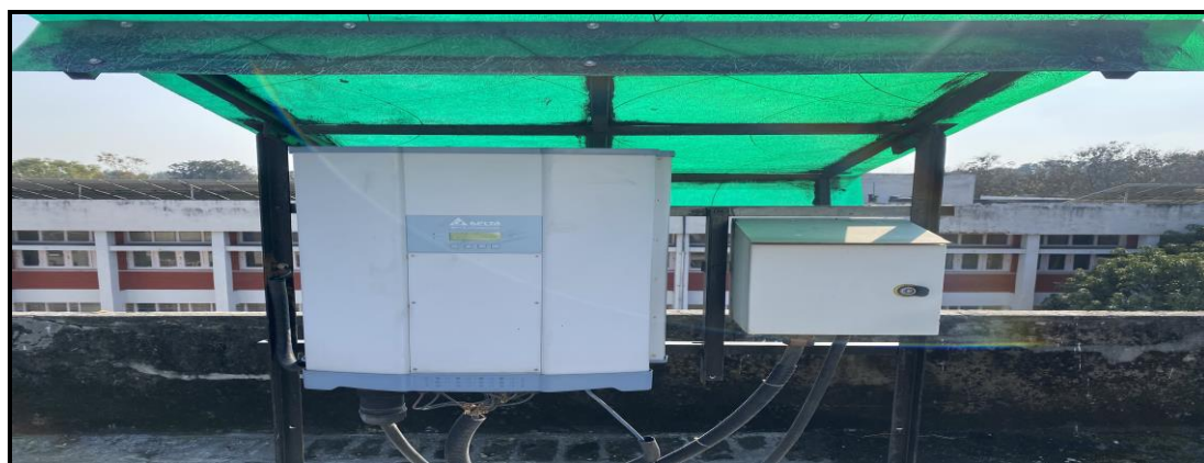
Solar Inverter at Different Buildings
